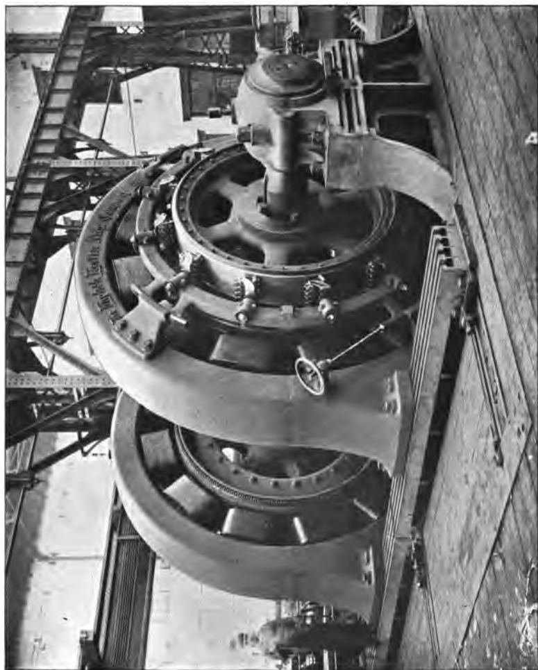
By permission of Dick Kerr and Co., London FIG. II. A TYPICAL ELECTRIC POWER GENERATOR—TWO DYNAMOS, EACH OF ABOUT 1,600 H.P.
